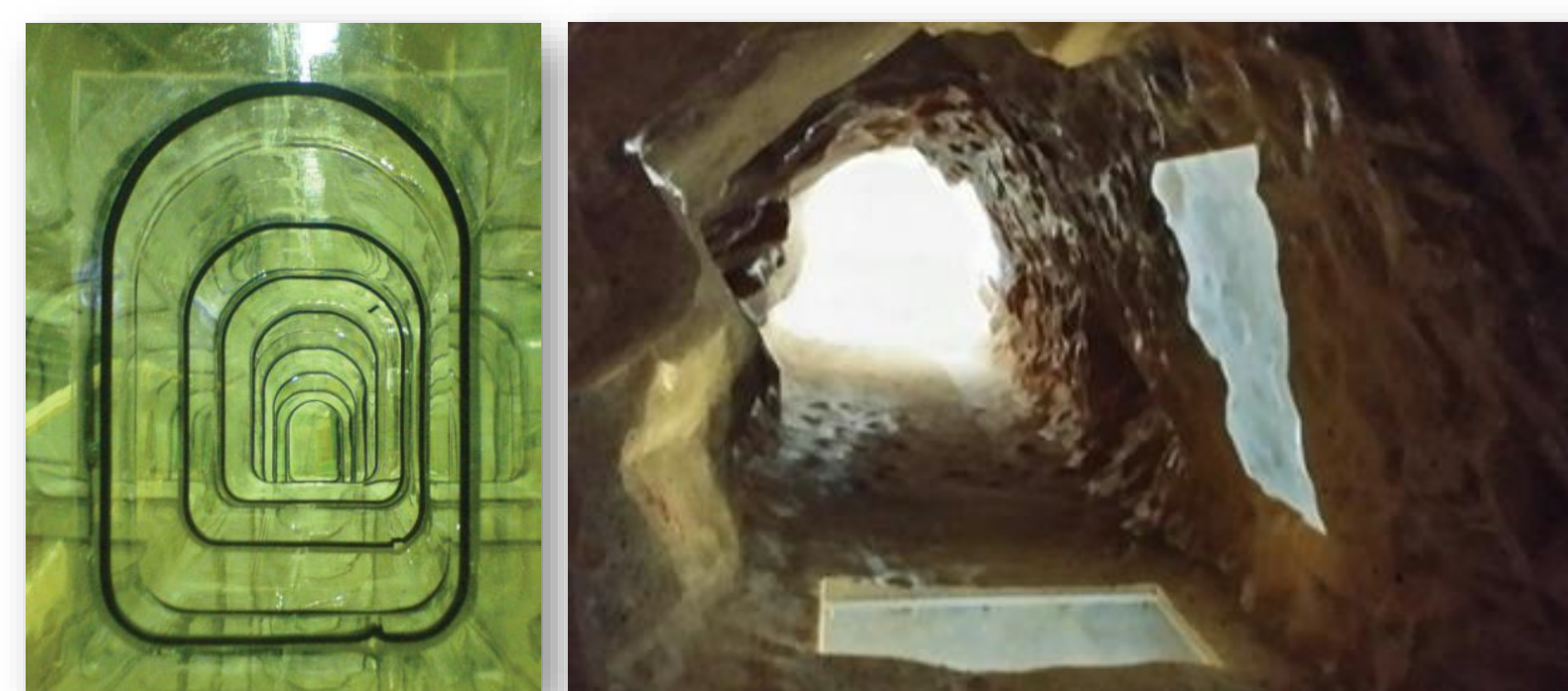
A classical model of an unlined tunnel and a view into a milled tunnel with access windows for optical flow measurements with Particle-Image Velocimetry (Potos: NTNU)
